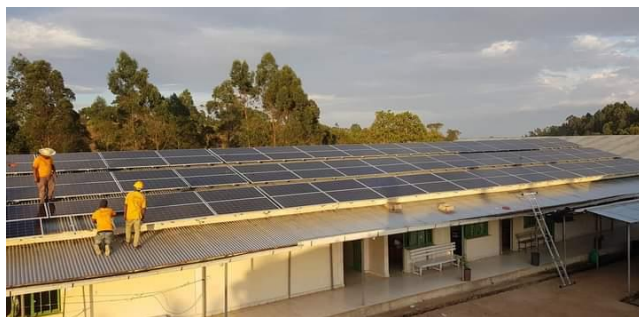
Figure 2. 6 Solar power system installation at Maji hospital
