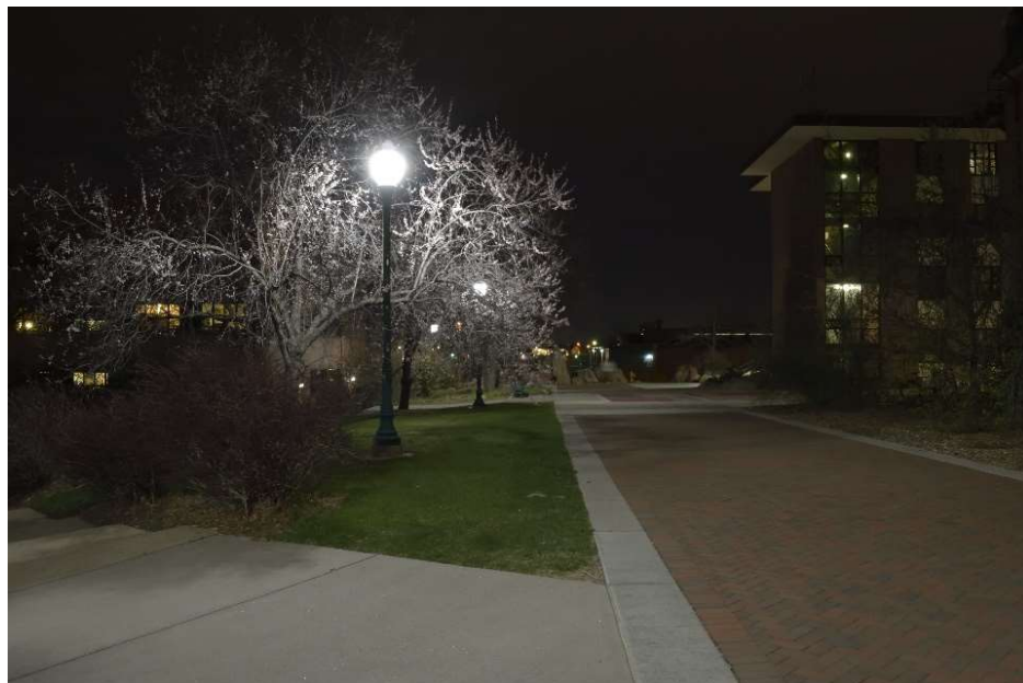
Figure 2: Acorn Luminaires near DeSmet and O'Connell Hall
