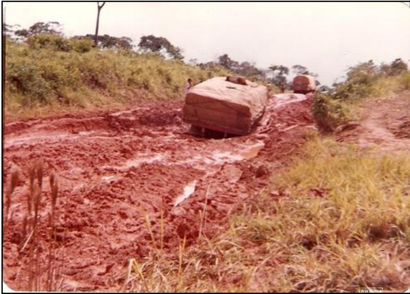
Figure 2.3 A photograph of BR-364 in 1984 shows just how difficult transportation was before the paving was complete (de Souza, 1984).
